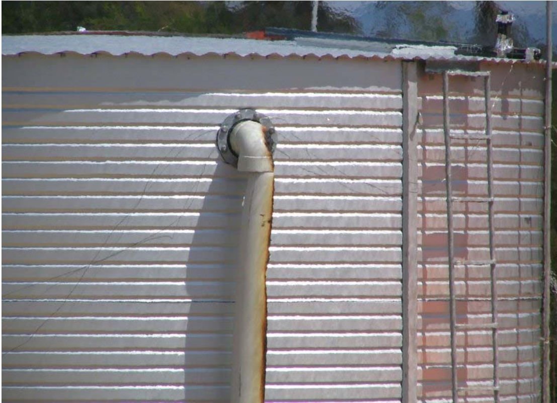
Figure C58 Bladder tank overflow charring during pre-radiation exposure.
