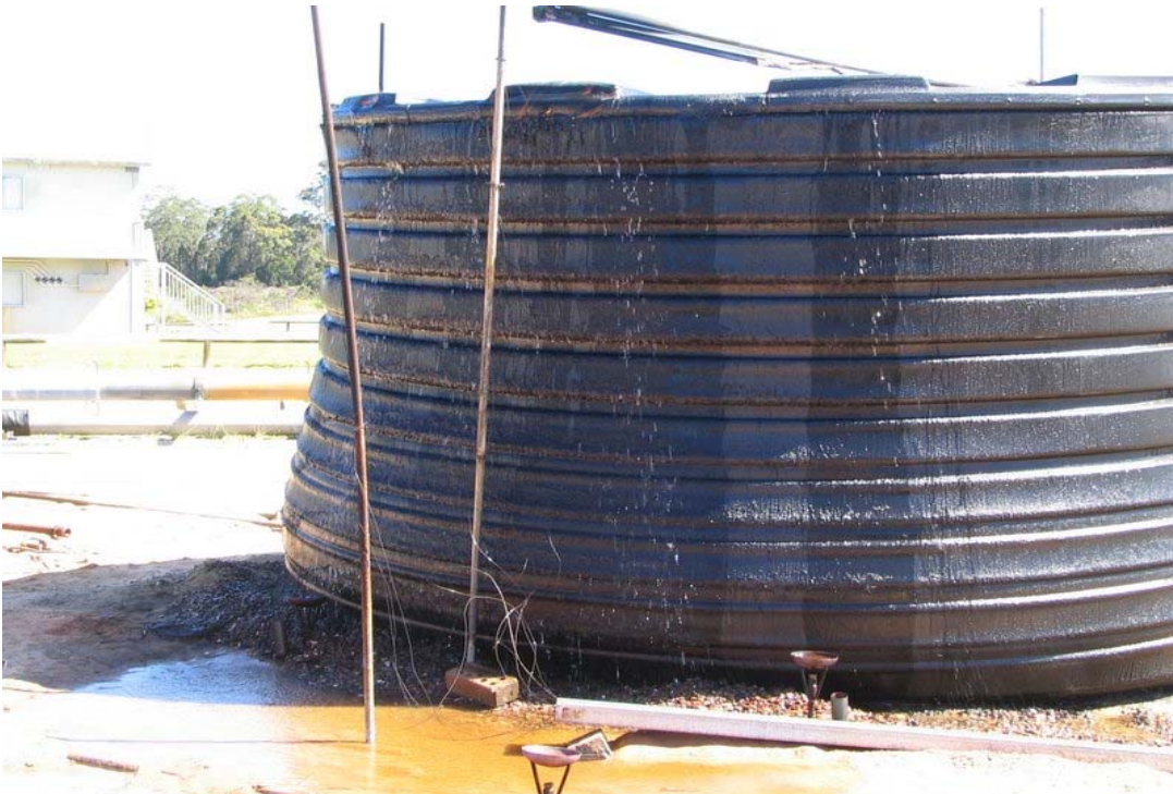
Figure C71 Tank 10 leaking as a result of litter ignition and pre-radiation exposure.
