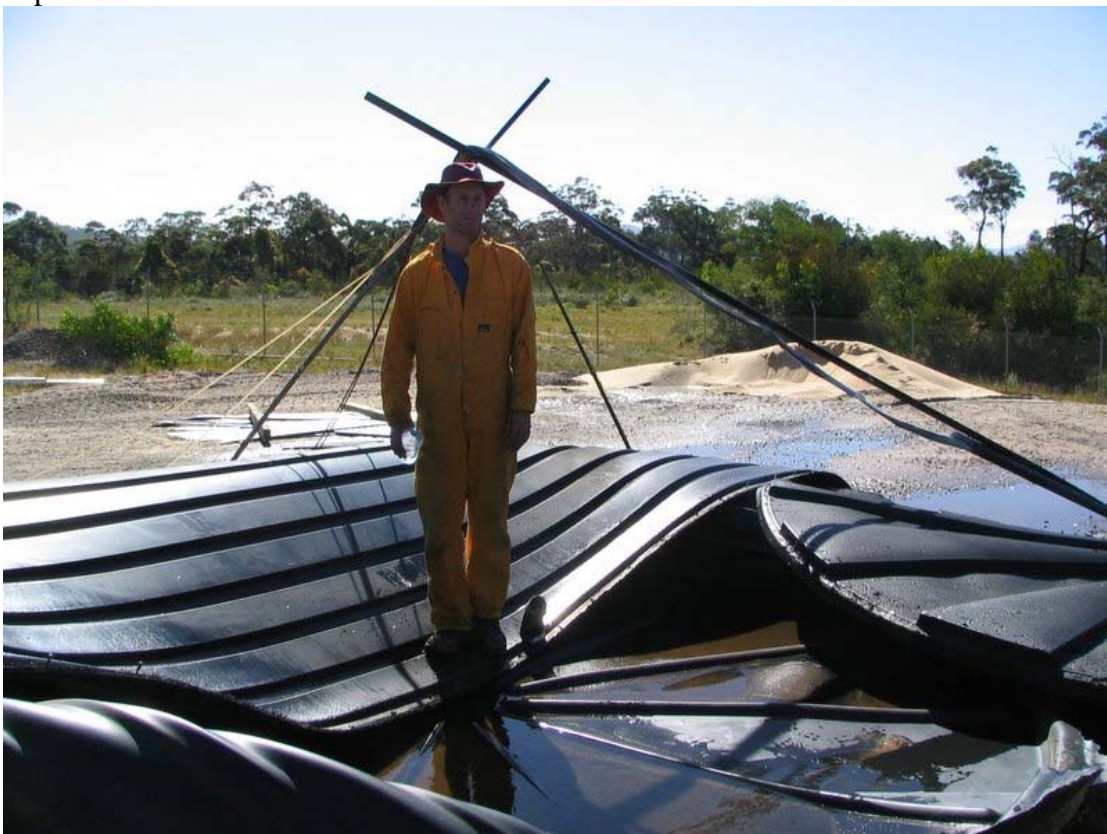
Figure C74 What remains of the completely destroyed tank 10.
