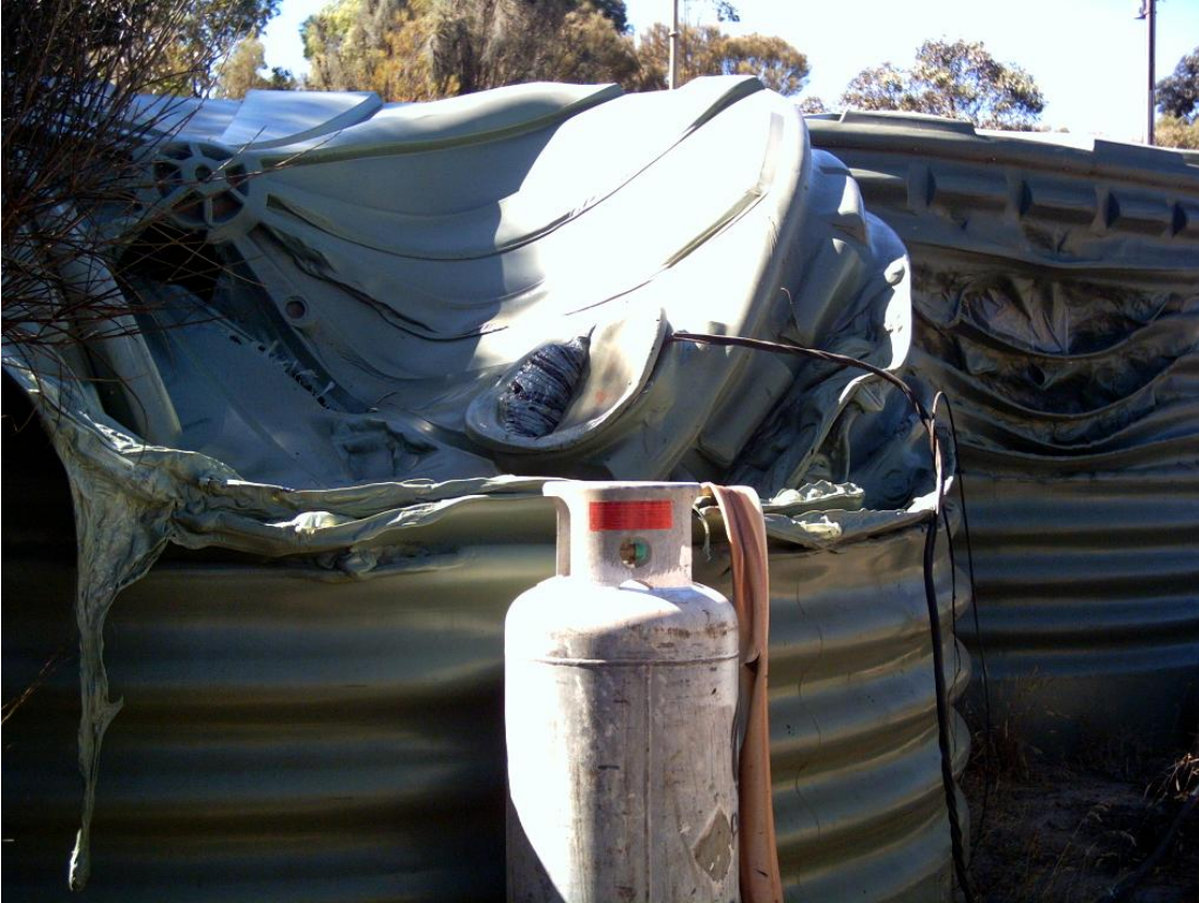
Figure 1 Example of water tank damaged, Eyre Peninsula
