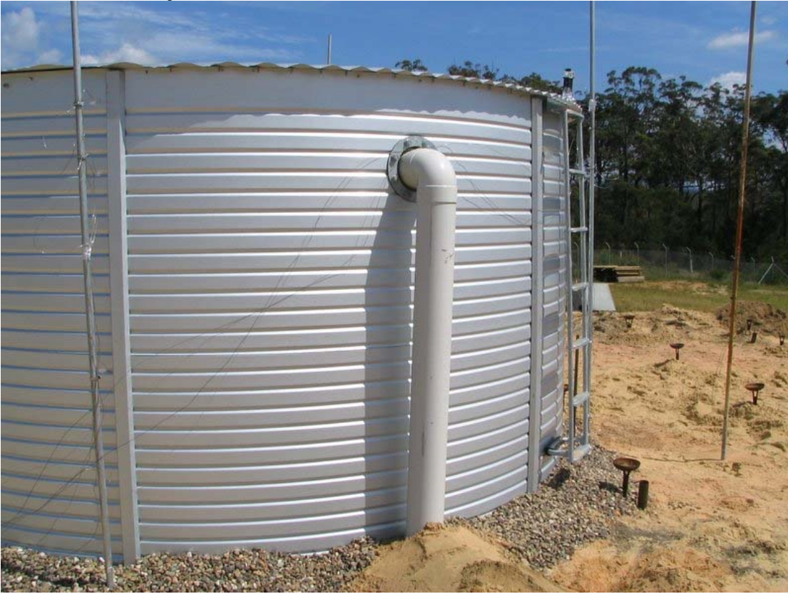
Figure C55 Tank 9, bladder tank.
