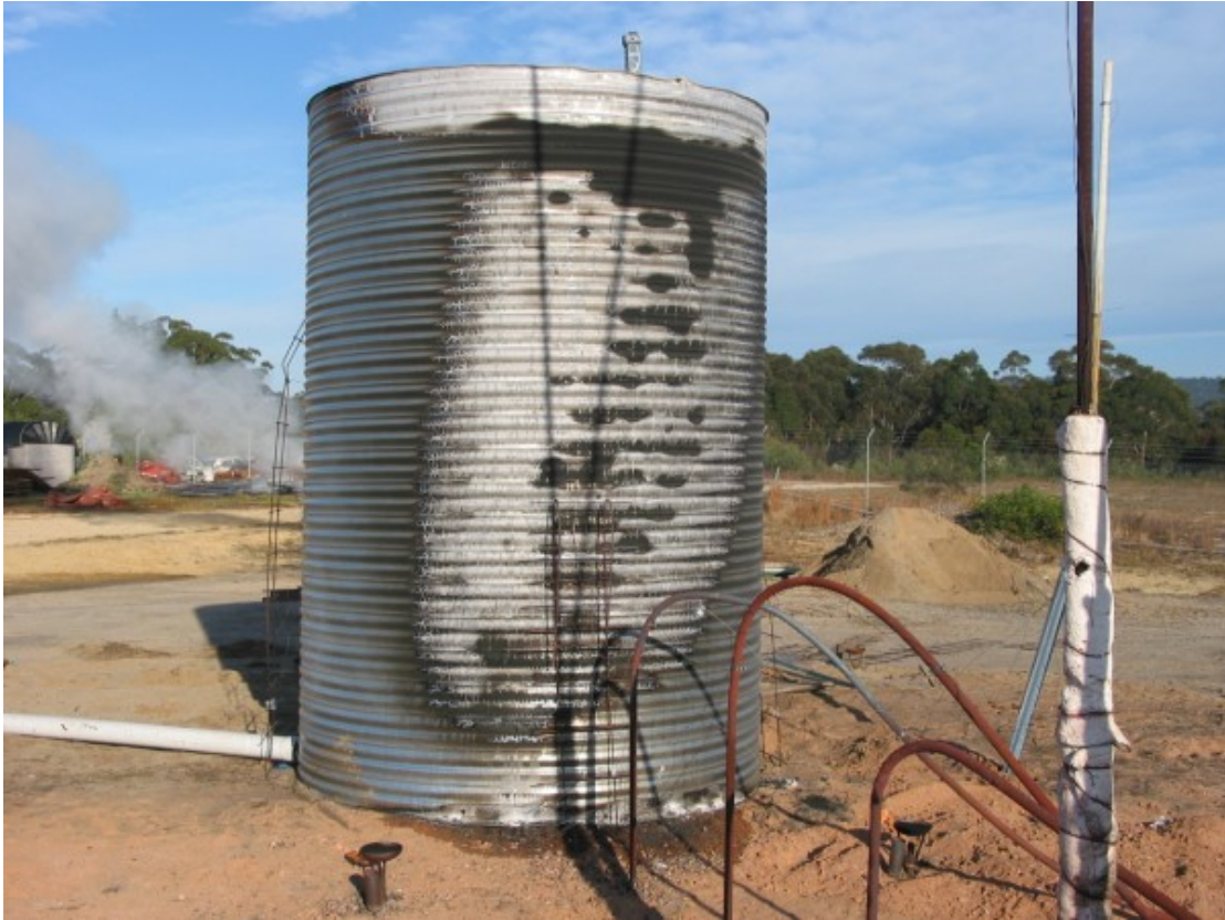
Figure C38 Tank 7 severe external damage resulting from structural exposure.
