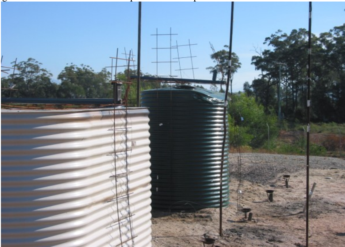
Figure C28 Tank two and four slight external damage resulting from pre-radiation exposure.
