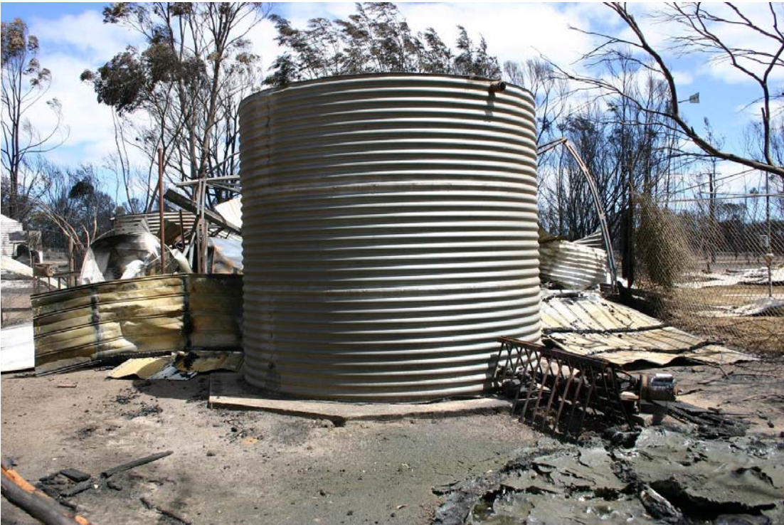
Figure 2 Example of metal water tank withstanding adjacent structure fire, Eyre Peninsula.
