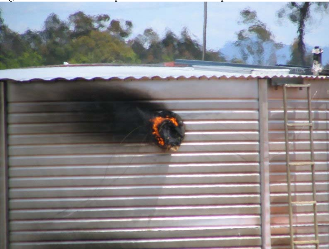
Figure C61 Damage to bladder tank overflow during pre-radiation and flame exposure.
